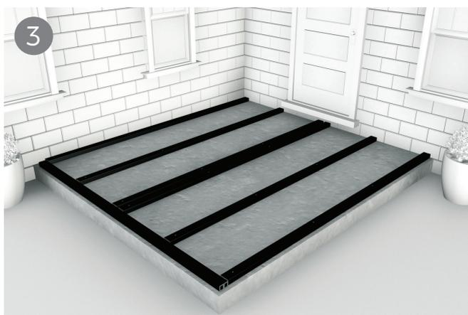
Step 3, The Structural joists can be secured down on every joist at both edges. With the joists spaced at 400mm this would mean approximately 18 screws per board.
